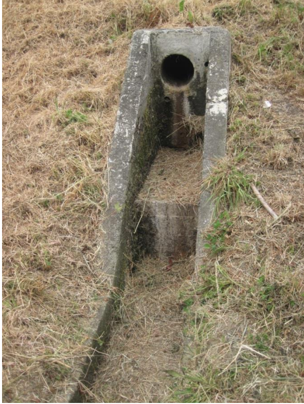
Figure 4-10: Narrow concrete channel from outlet to stream
