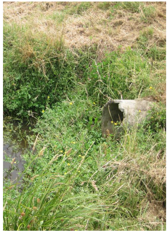
Figure 4-7: Protruding outlet
