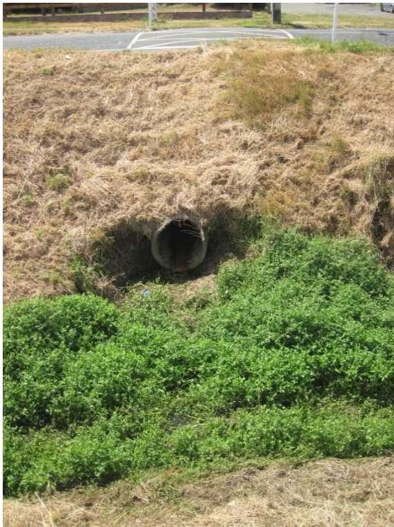
Figure 4-6: Protruding outlet
