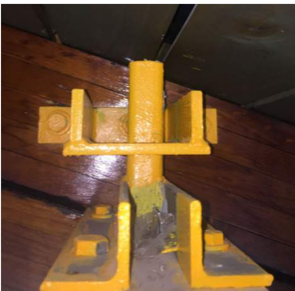
Figure 4.1 – Glazed End wall top connection with little to no travel room
