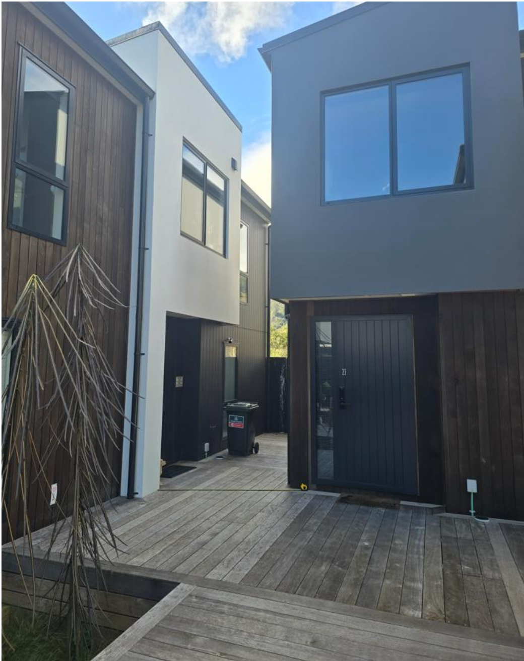
Figure 4: "Tee" dead-end section with approximately 1.8m wide access.
