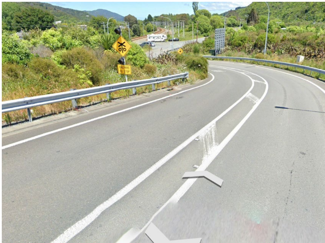
Figure 6-2: Manor Park Road/ Benmore Crescent intersection Sightline
