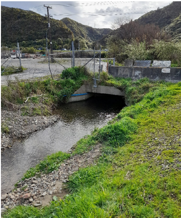
Figure 3-3 Outlet of culvert 1
