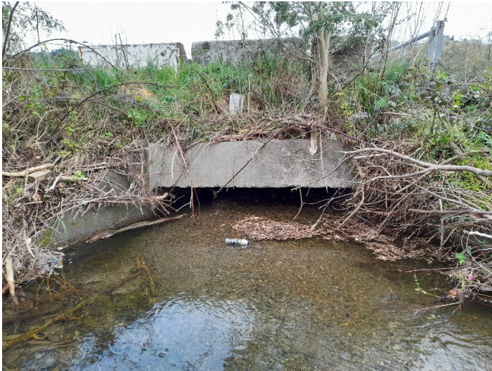
Figure 3-2 Inlet to culvert 1
