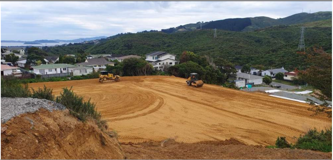
Photo 1 – Bulk Filling – MSE Wall 05
