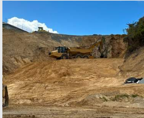
EW02, approximately half completed
