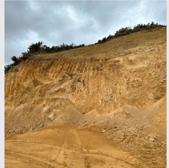
Grading of the slope at the northern extent of EW02.
