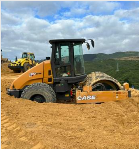
Broken down roller.
