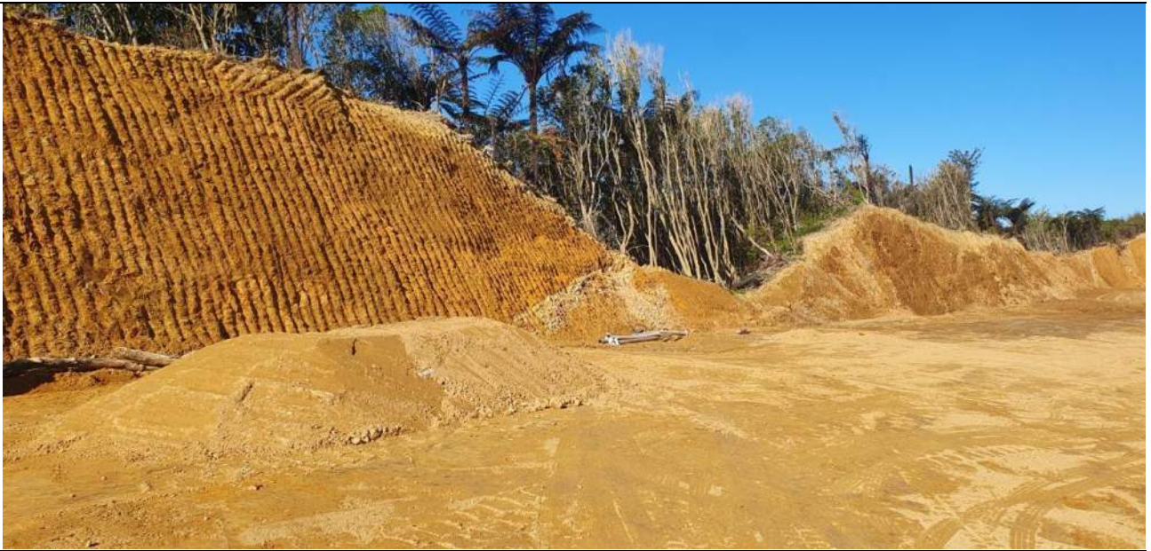
Photo 3 – Temporary cut slopes at Stage 6
