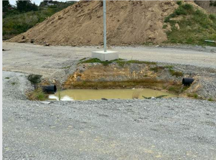
Intermediate pit for silt sedimentation.
