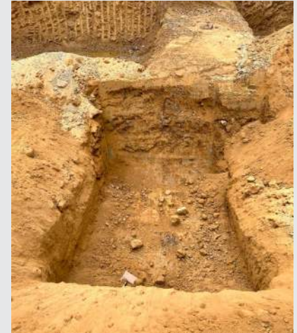
Excavated area at the back of the toe
