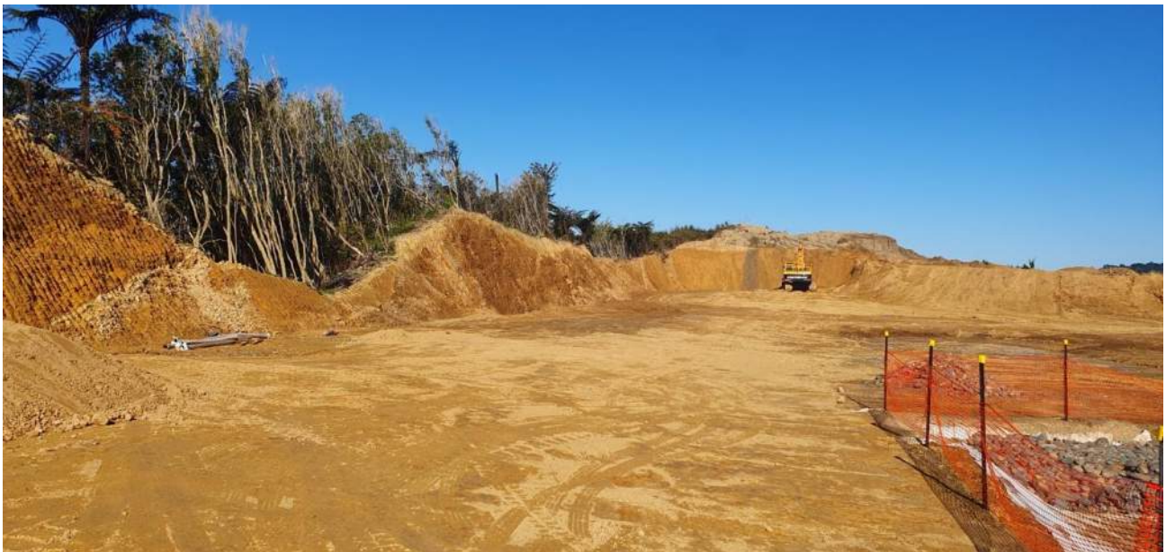
Figure 2: Bulk cutting showing insitu Greywacke across the level platform
