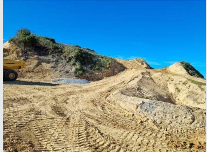
EW02 - Looking south-east, showing the tie in of the shoulder of the MSE wall into the existing ground level.
