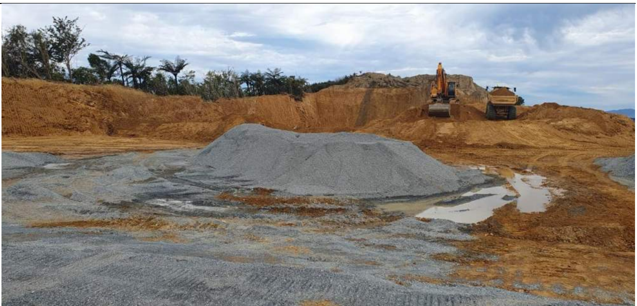
Photo 2 – Stockpile of GAP40, placed as capping for winter, Stage 6. In the background, bulk cutting for placement of fill at MSE Wall 05
