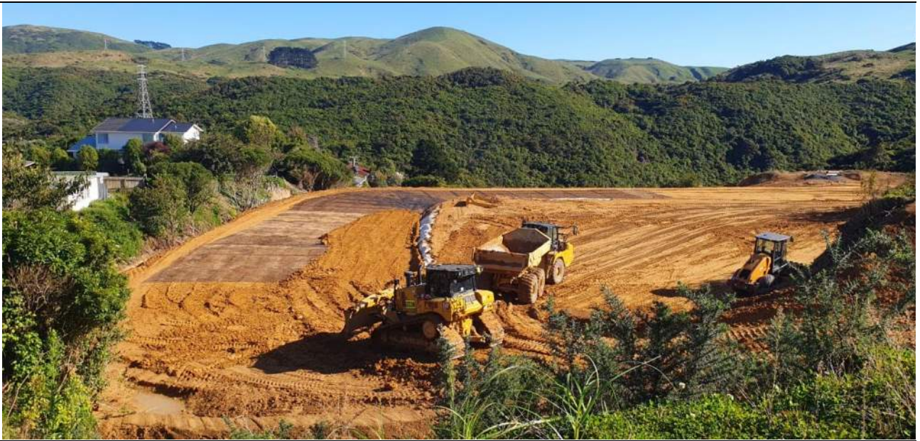
Photo 1 - Bulk Filling - MSE Wall 05
