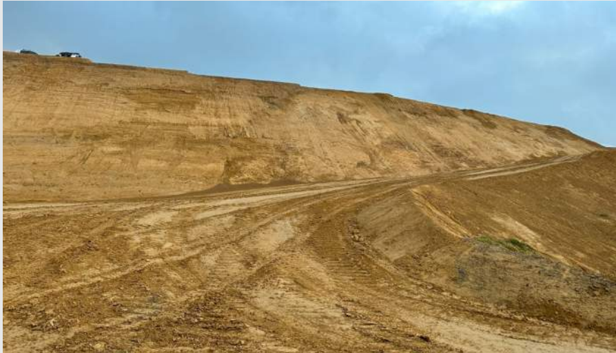
EW02 and 45 degree cut slope extending to the south
