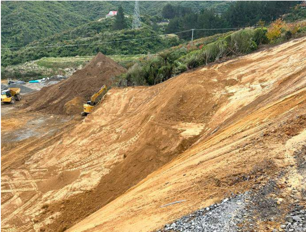
Figure 1 – Current status of the bulk cutting to the north of EW 02.
