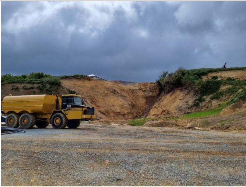
Photo 1 –EW 02, on hold pending receipt of final designs
