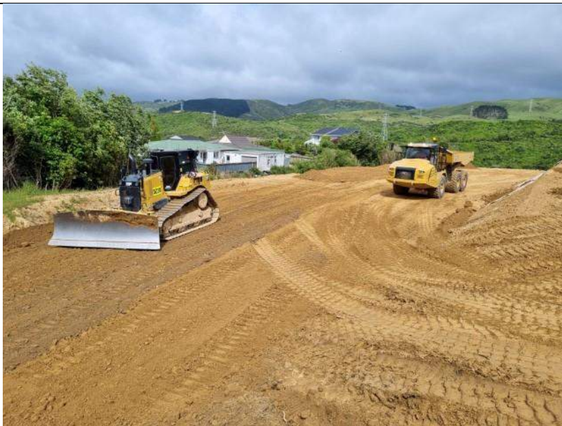
Photo 2 – Blading out bulk fill for EW 05
