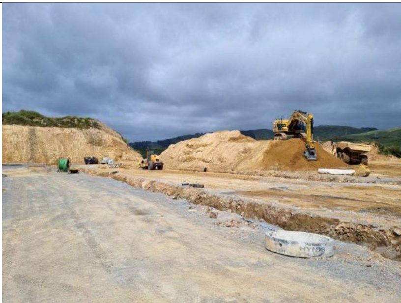
Photo 4 – Stockpile source material carting to EW 05
