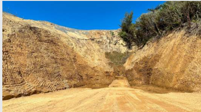
Excavation backfilled to target height. Saturated areas from ephemeral stream visible.
