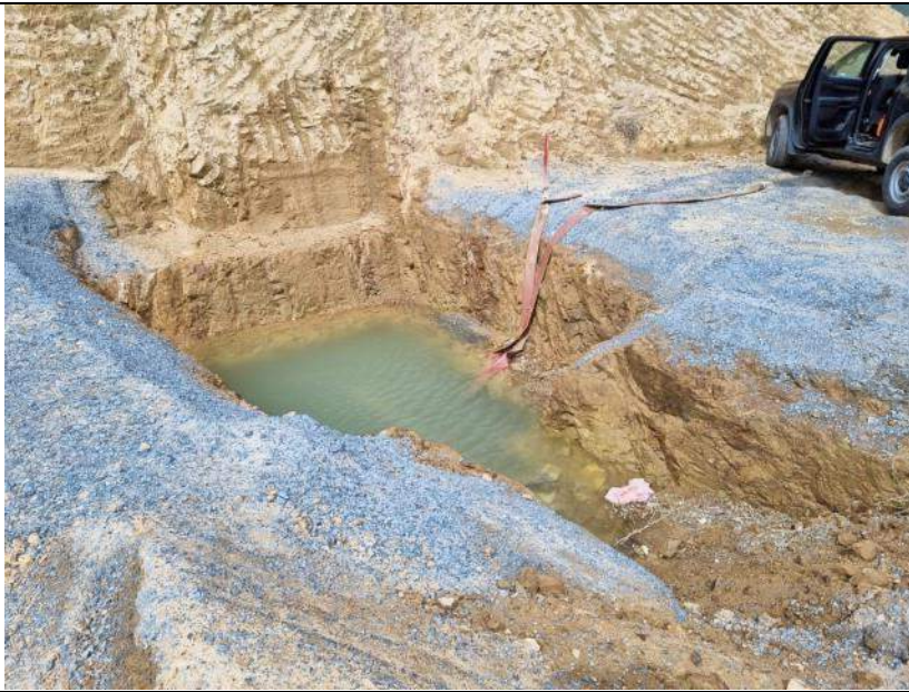
Photo 3 – Sediment detention basin, for pumped surface water
