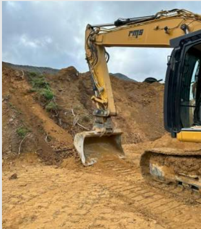
Extending subsoil drains.
