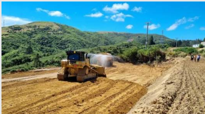
Blading out the structural fill to EW 05
