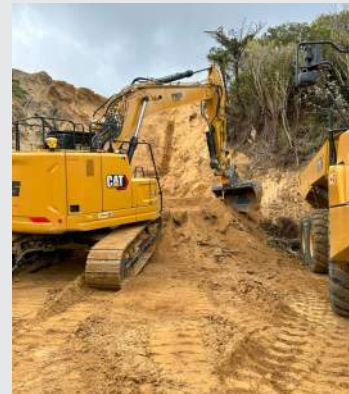
Trees and organics being cleared
