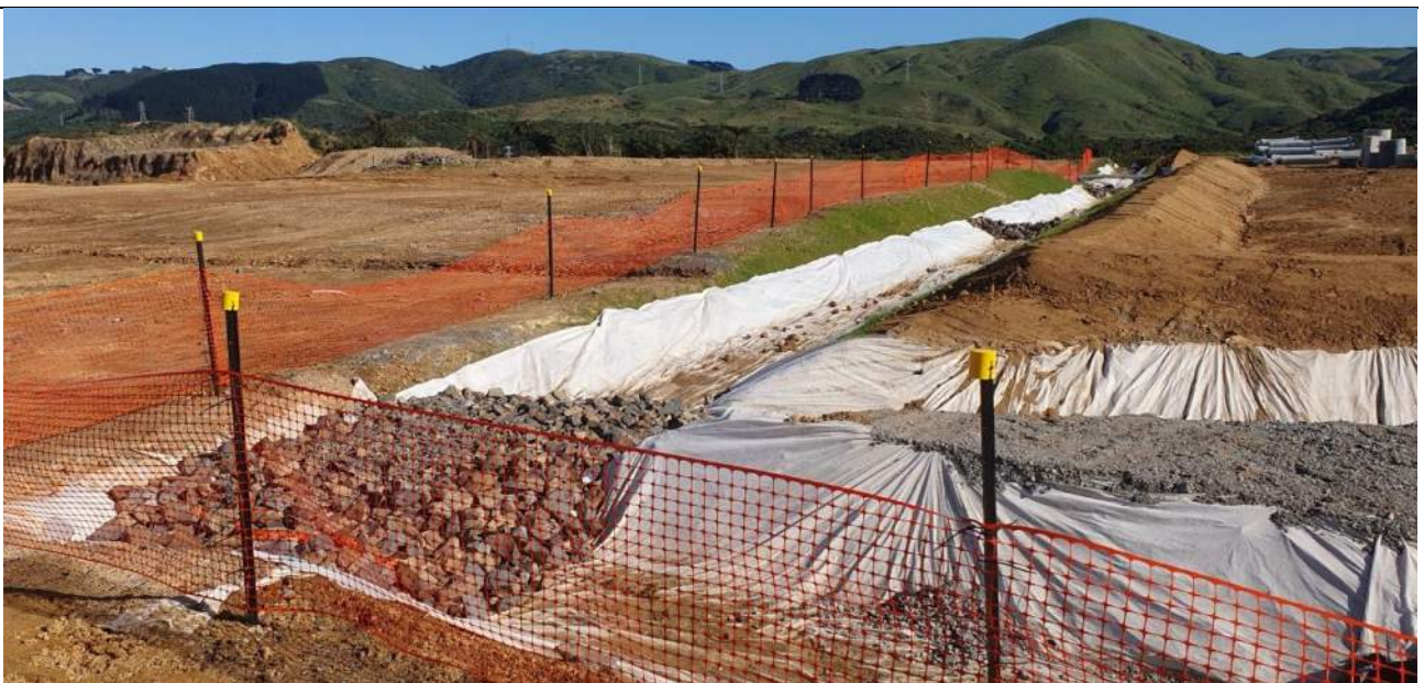
Photo 2 - Sediment containment/treatment devices
