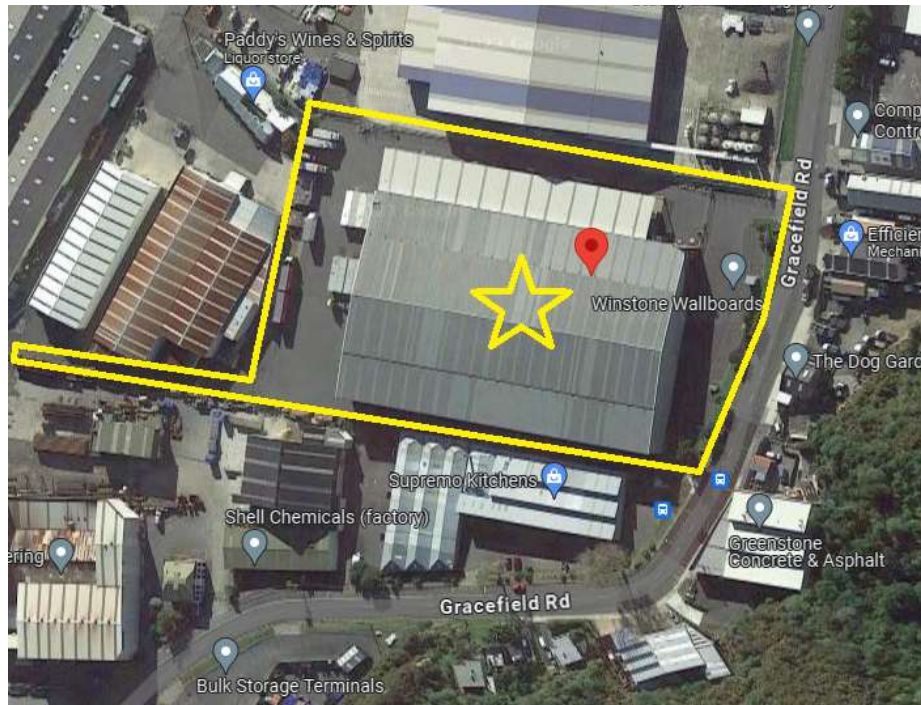
Figure 1: WWB's Gracefield site, outlined in yellow and indicated by a yellow star. Source: Google Maps, annotated by RMG, March 2025
