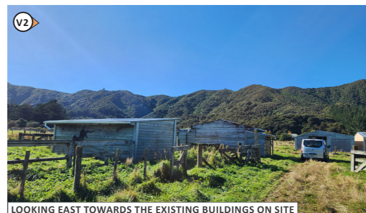
LOOKING EAST TOWARDS THE EXISTING BUILDINGS ON SITE
