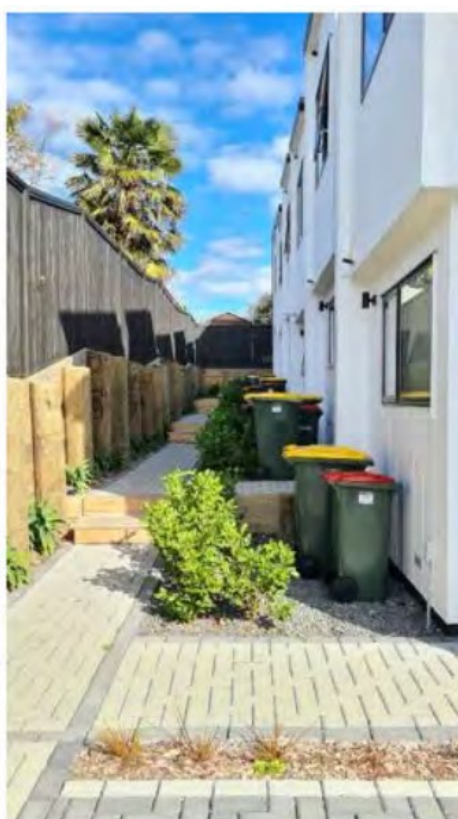
Figure 3: Bins areas without screens and stair access.
