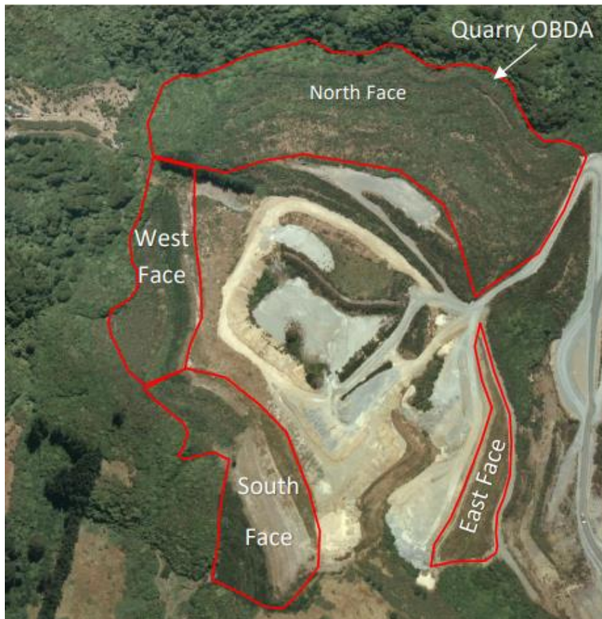
Figure 3: Domains of the overburden disposal area. The process void is in the centre. February 2019 photographs. Source: Tonkin + Taylor Geotechnical Assessment.
