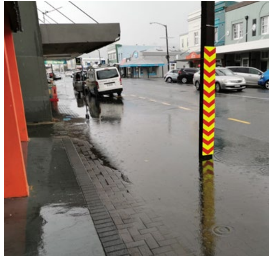
Current flooding during wet weather - Jackson Street
