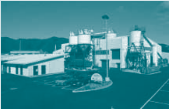
Seaview Wastewater Treatment Plant
