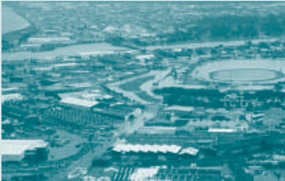
Flood damage caused by recent flooding
