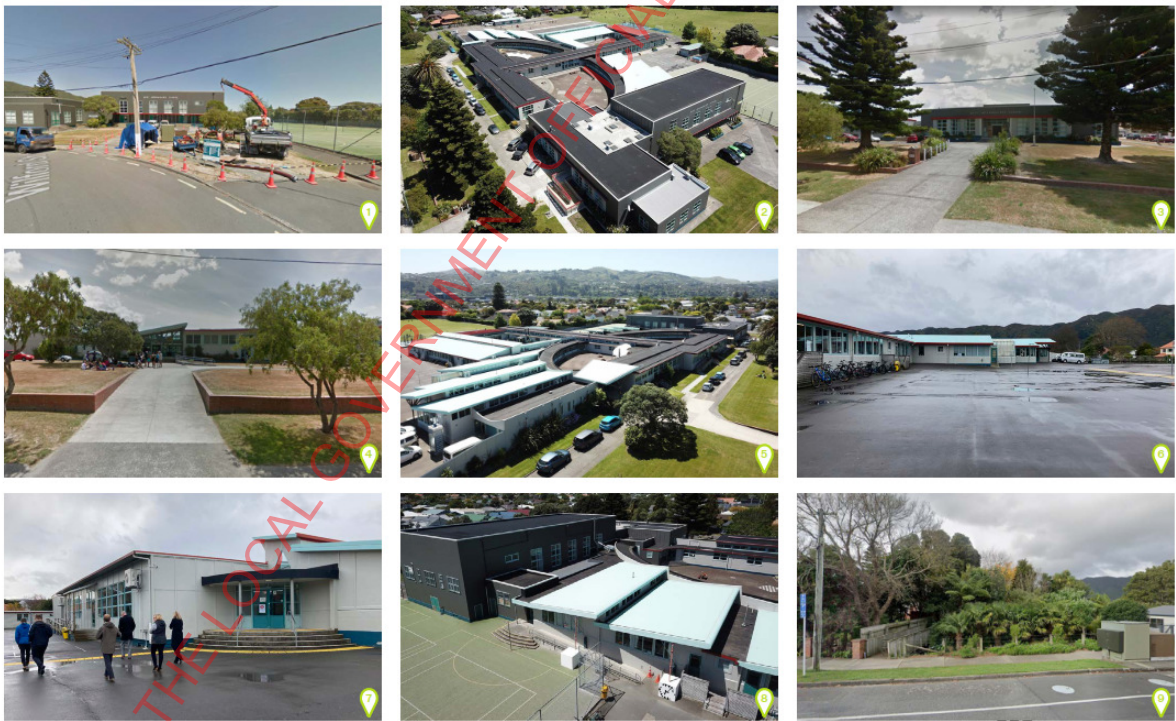
Figure 4: Site Photos - JASMAX Architecture
