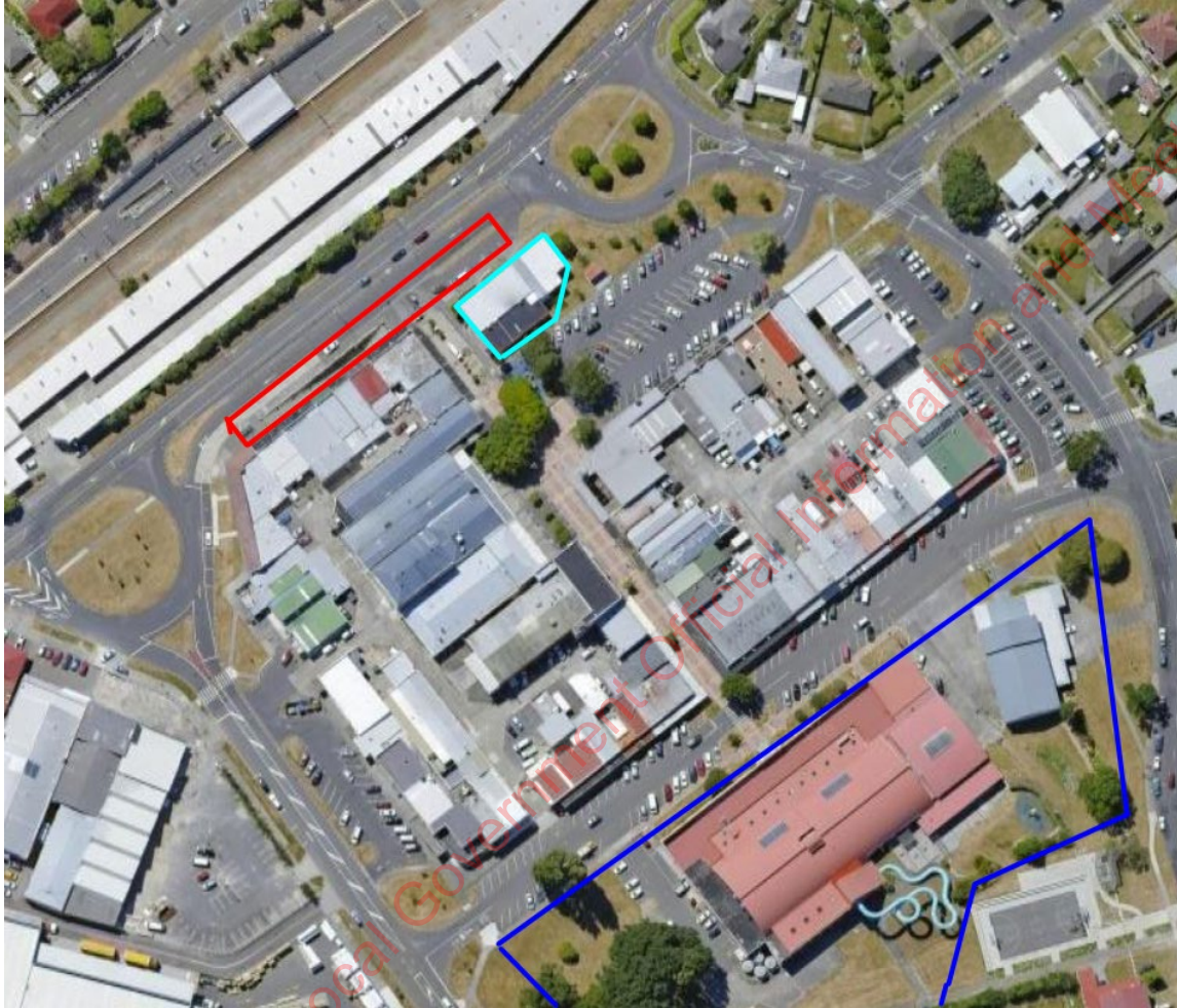
Ref 1 Overhead View of Hillary Court and Surrounding Streets
