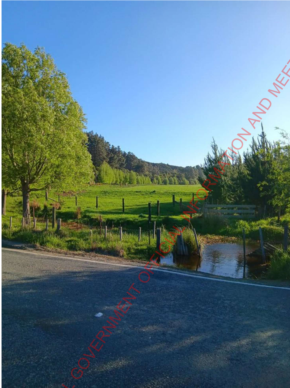
Figure 6: Culvert feeding Wetlands from 915 with Fill site in background
