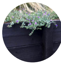
Square timber retaining wall
