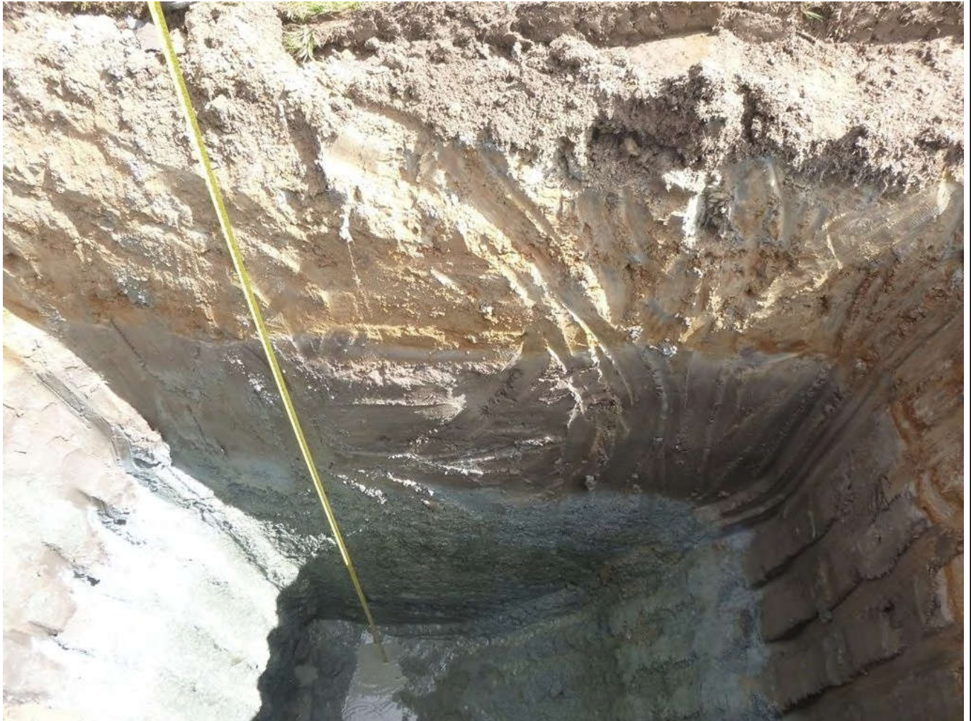
TP01 - western face of trial pit 1
