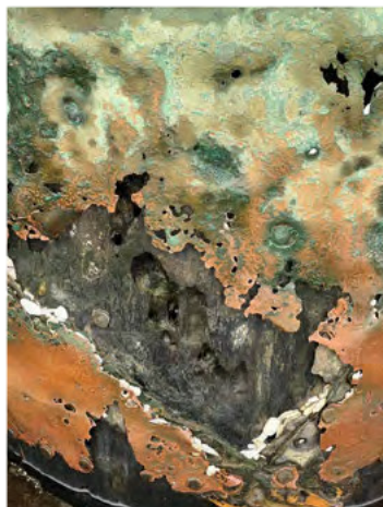
Figure 9: Failed copper sheathing and worm damage
