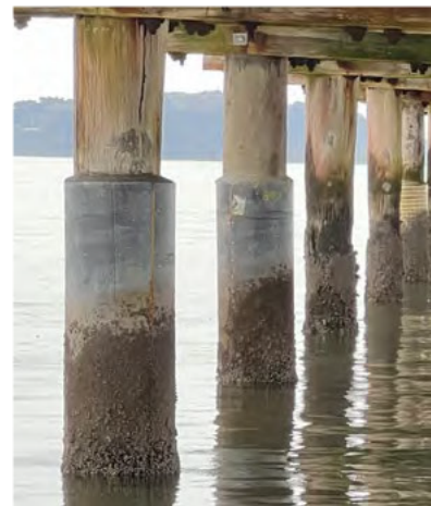
Figure 10: Piles with FRP jackets at Petone Wharf
