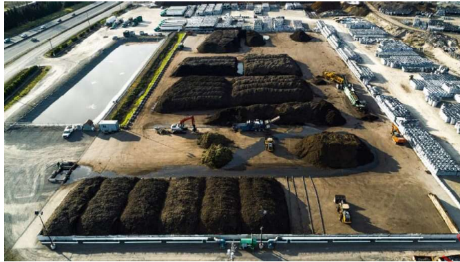
Photograph Appendix C.5: Aerated Static Pile Composting Operation.
