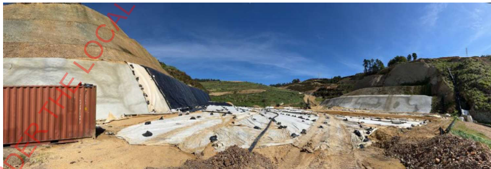
Image 1: Construction works for the new Phase 3
