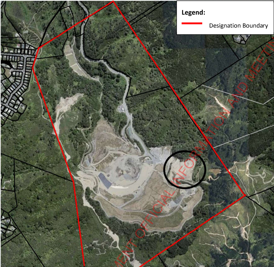
Figure 2.2: Aerial view of site and location of proposed works in black circleCopyright TTMapView 2024
