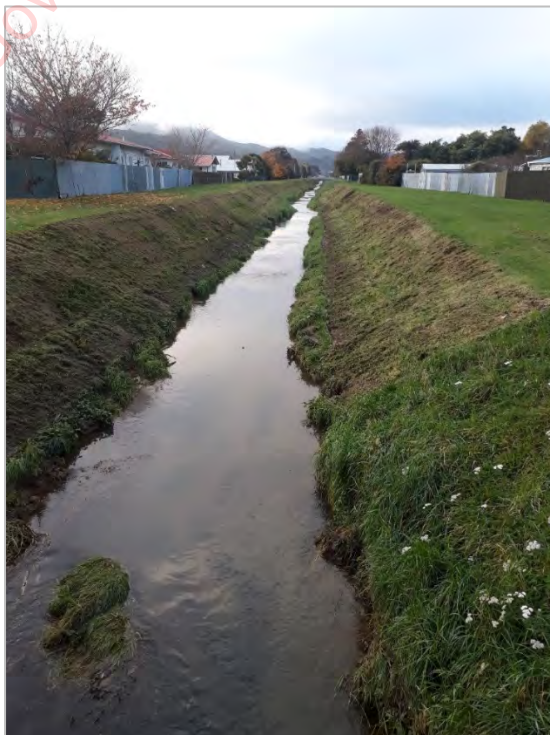
Figure 7-11 Black Creek looking upstream from Nelson Crescent Bridge
