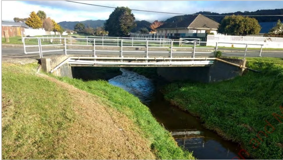
Figure 7-9 Norfolk Street bridge
