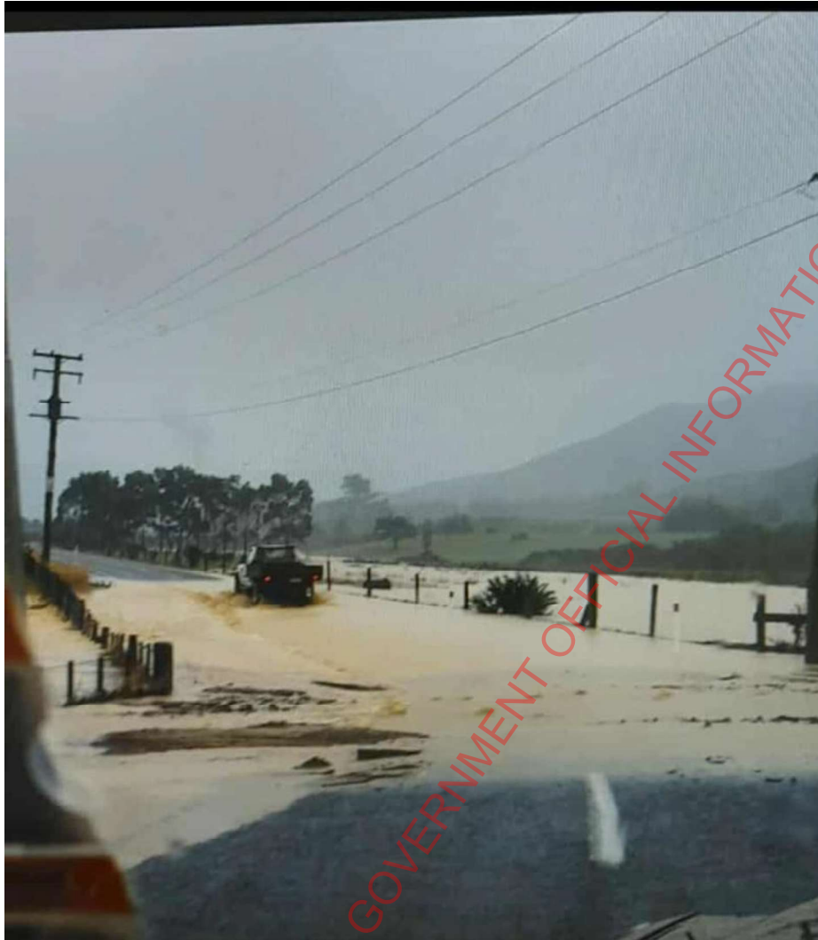
Photo of the need to keep the spillway open so that residents don't get trapped down Coast Rd (taken in 2022)
