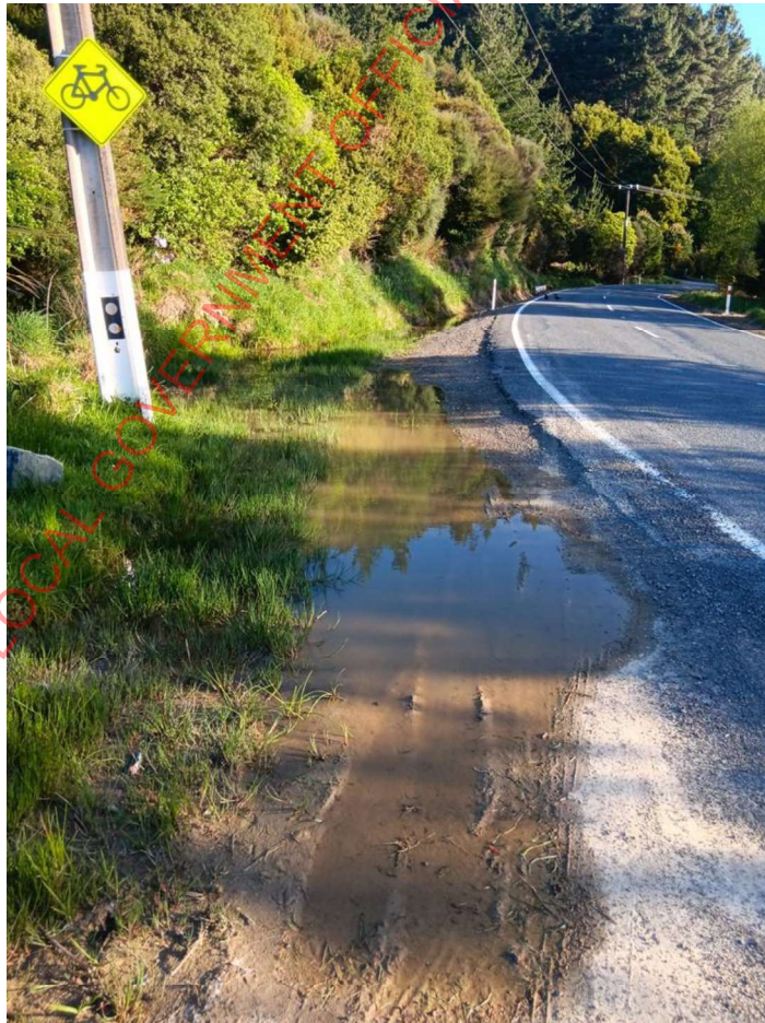
Figure 9: Flooding from 915 Wetlands
