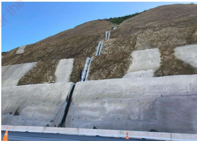
Figure 7 Example of re-profiling and benching
