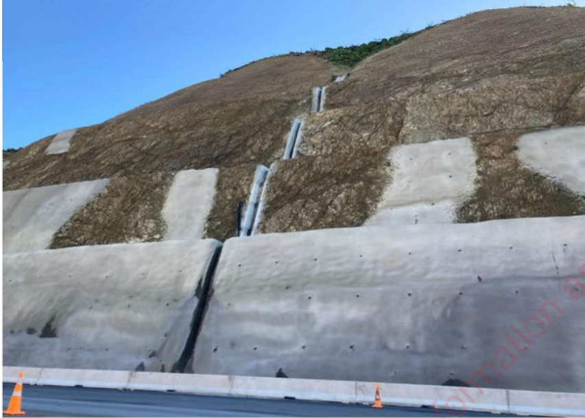
Figure 7 Example of re-profiling and benching
