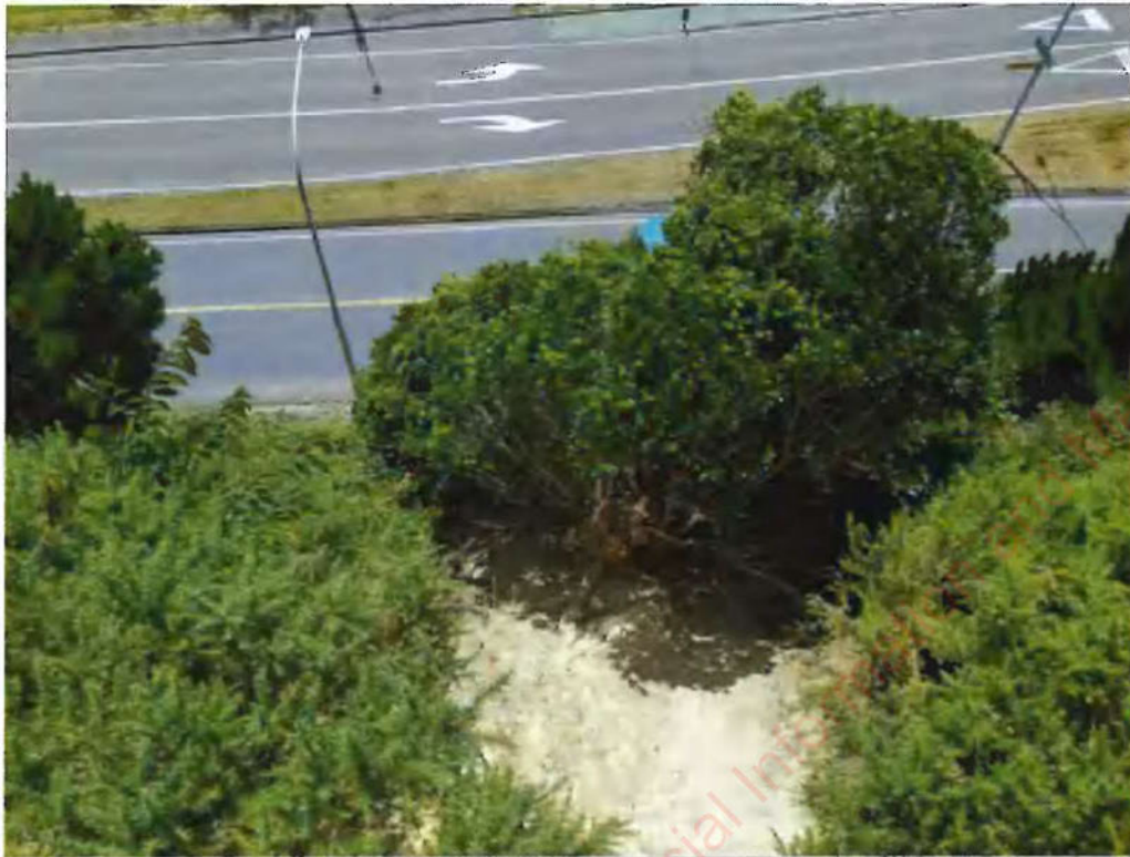
Photograph 3: View of landslip 1 from above – taken from deck (Photo taken 10 January 2022).
