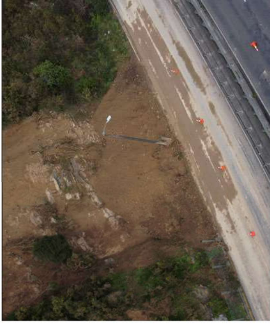
Figure 7 Aerial view of the Eastern Hutt Road
