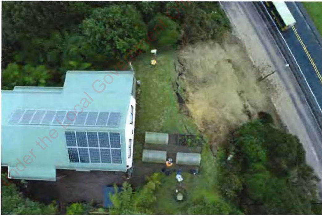
Photograph 6: View facing directly down from above, showing landslide headscarp. Taken 26 July 2022.
