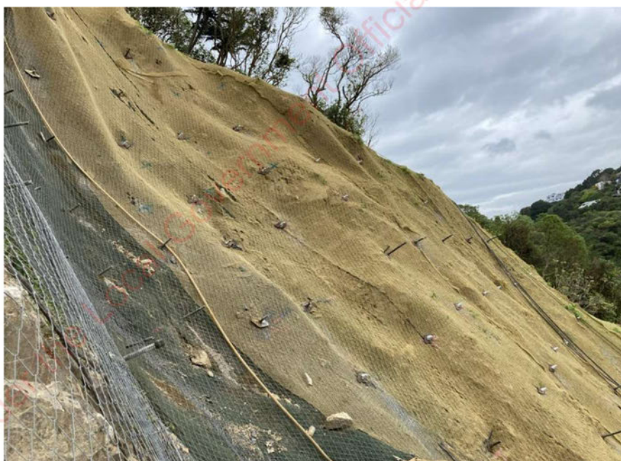
Figure 5 Example of pinned erosion control matting
