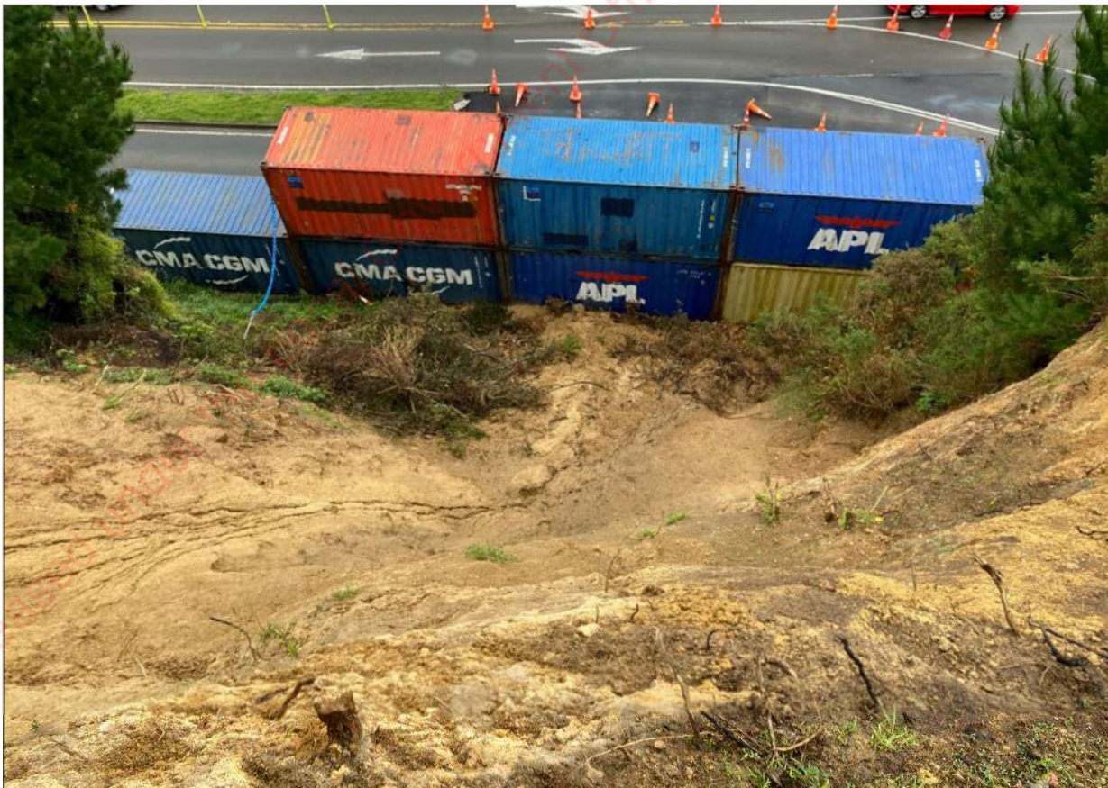
Figure 2 View behind the containers following completion of the temporary works
