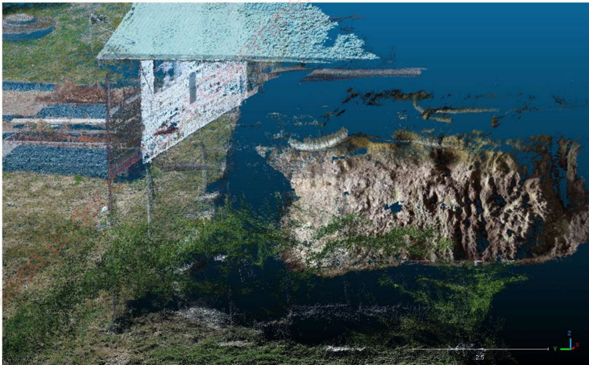
Figure 3 Point cloud - excavation for house foundations
