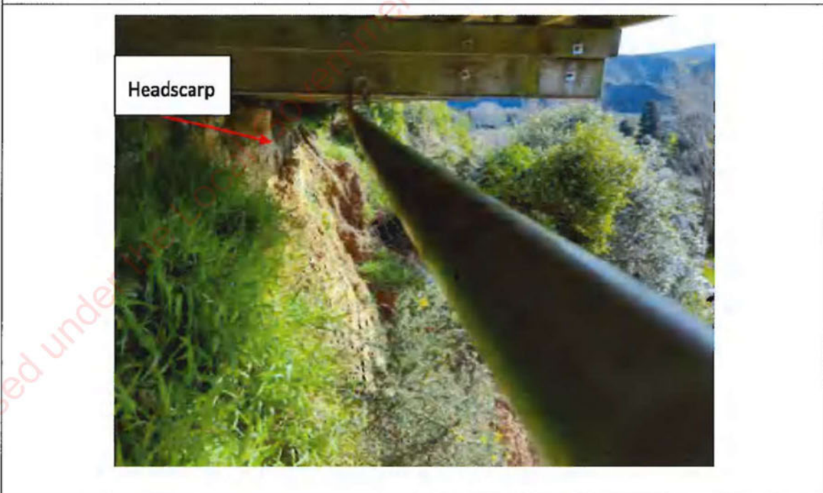
Photograph 8: View at top of landslide 1 from below deck (looking from east to west) (Comparison photo taken 23 August 2022).
