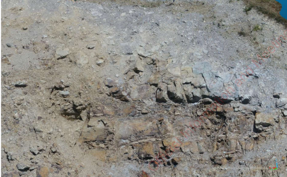
Figure 5 Rock exposed in slope, below and adjacent to view in Figure 4
