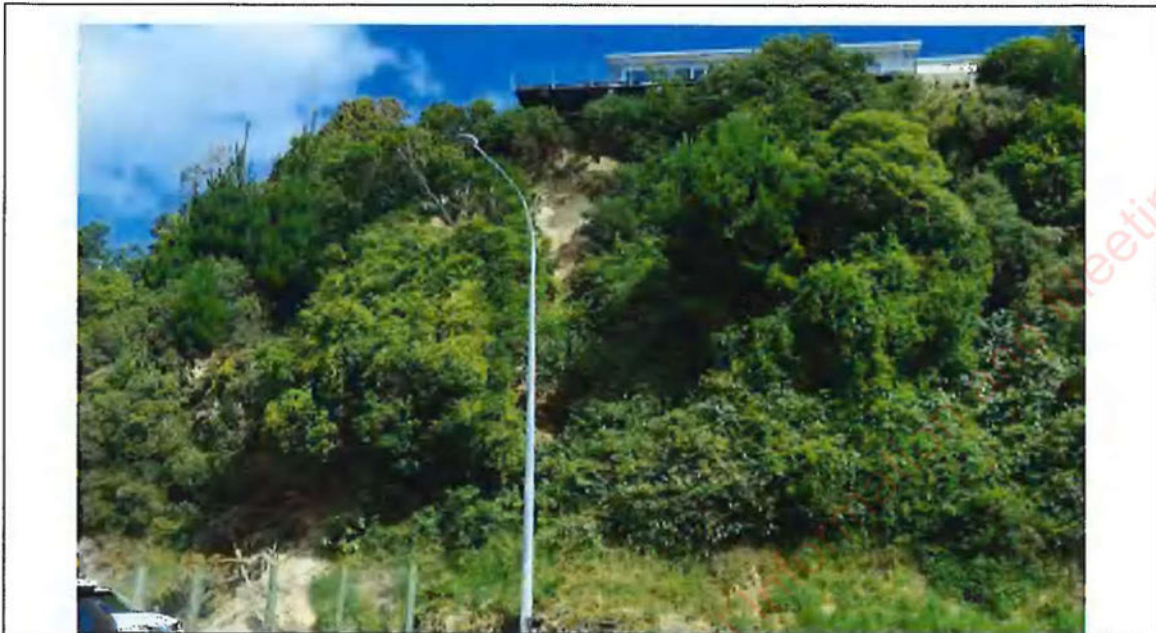
Photograph 1: Dwelling and landslip 1 from Eastern Hutt Road (Photo taken 10 January 2022).
