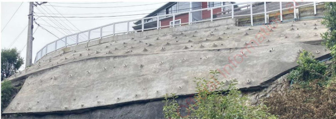
Figure 6 Example of anchored shotcrete
