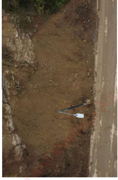
Figure 10 Debris accumulated along the shoulder
