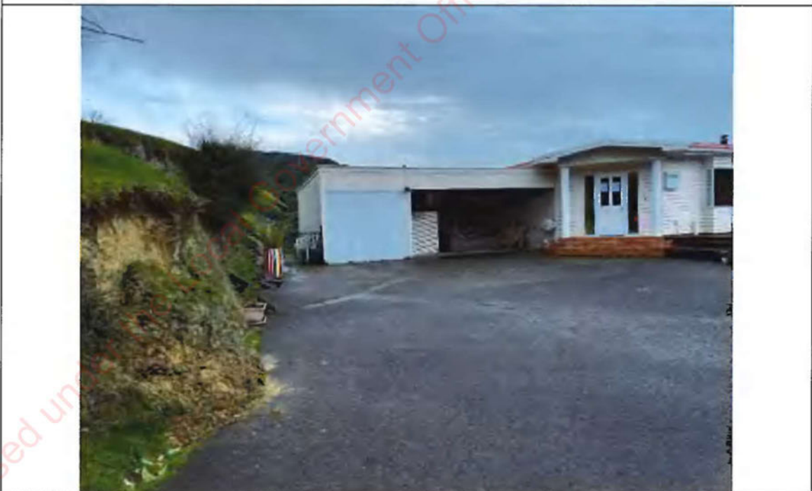
Photograph 20: Landslip 2 taken looking north with dwelling in background. (Photo taken 26 July 2022).
