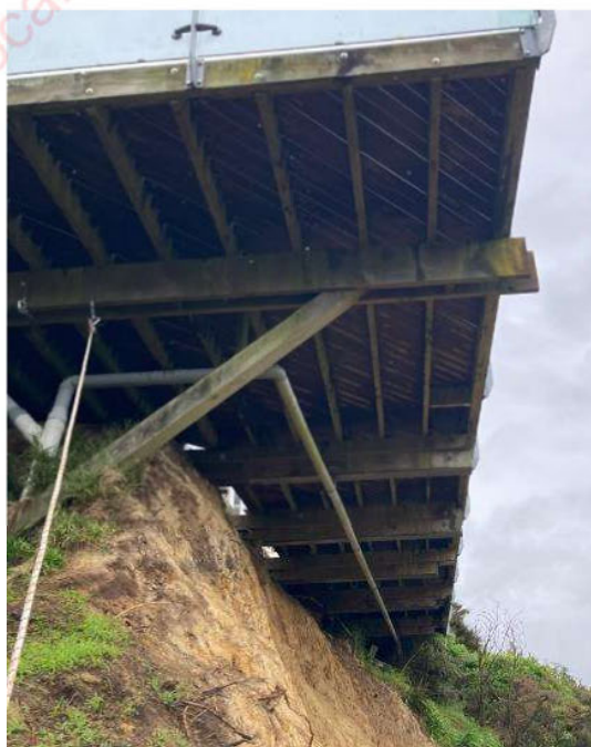
Figure 3 View of cantilevered deck and proximity of existing instability
