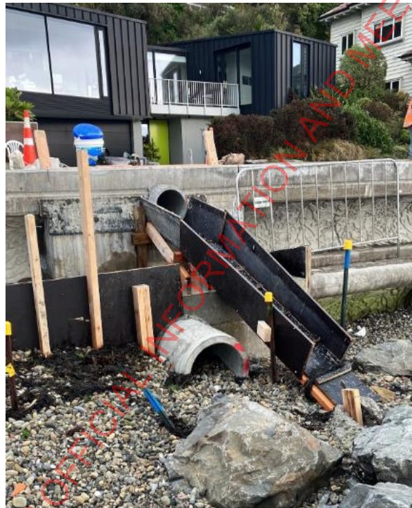
Figure 5.3: Wooden ramp / stairs to allow kororā to access the culvert
