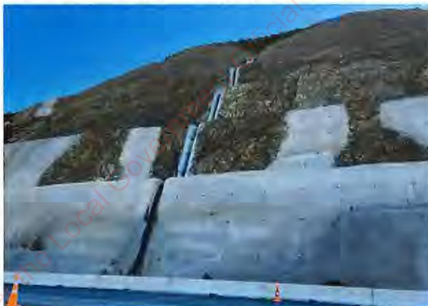
Figure 4 Example of re-profiling and benching
