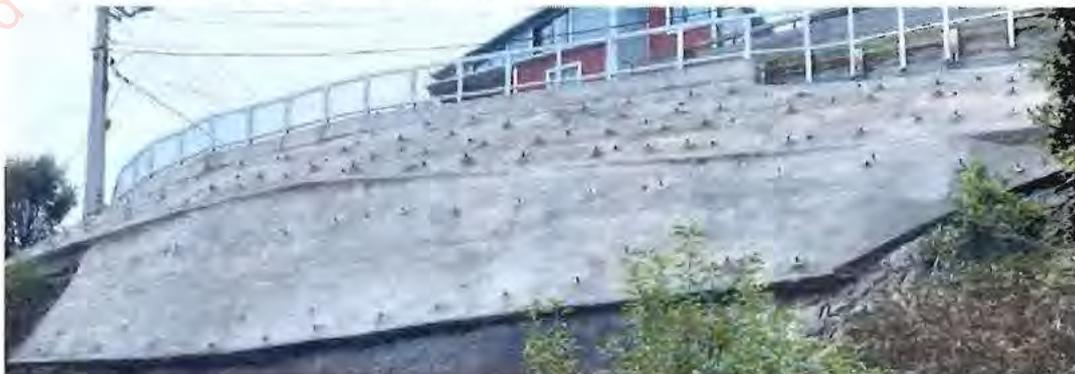
Figure 3 Example of anchored shotcrete
