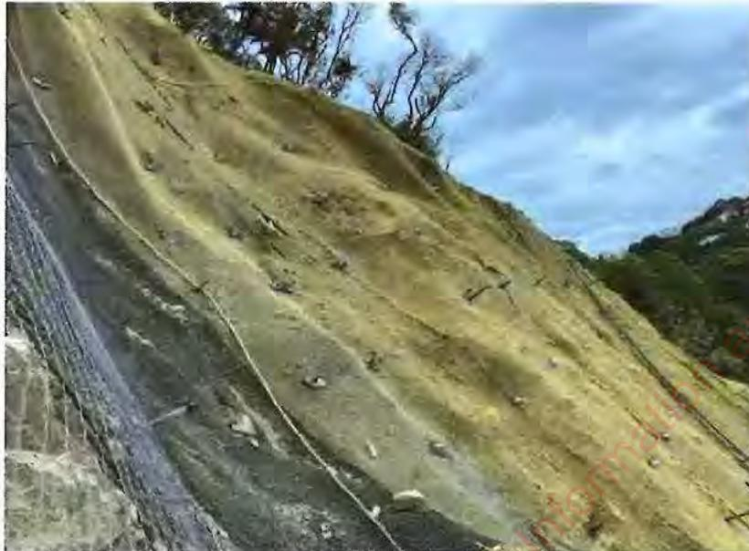
Figure 2 Example of pinned erosion control matting
