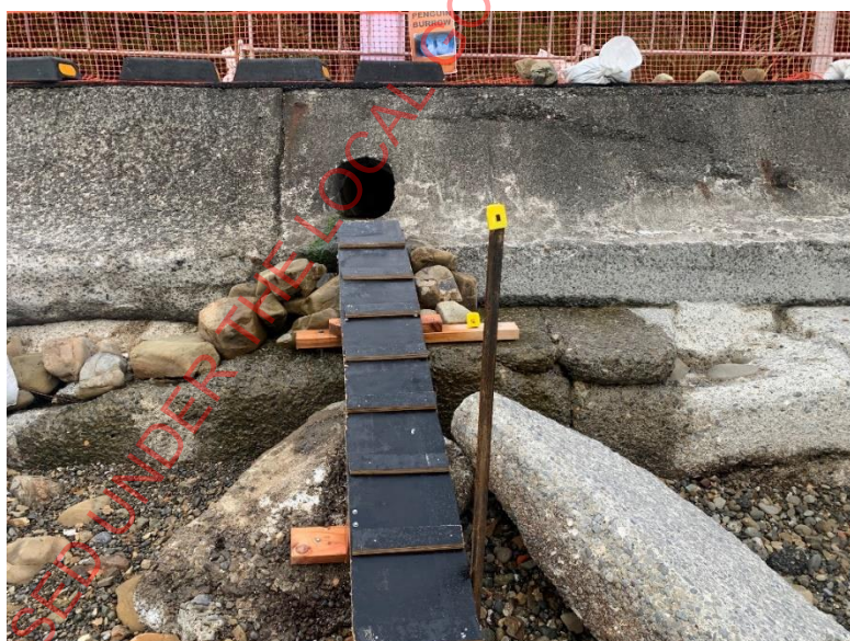
Figure 6.2: Wooden ramp / stairs to allow kororā to access the culvert
