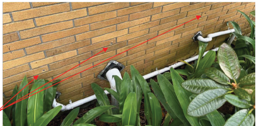
Right: Drill bore anchors still present in wall. More possibly present.
