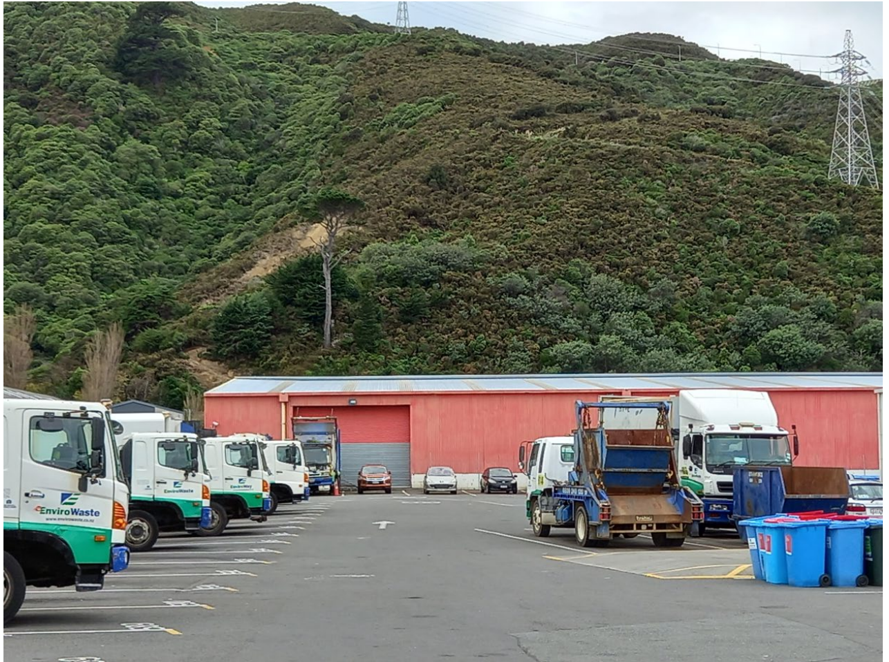
Figure 1: Gracefield depot site
